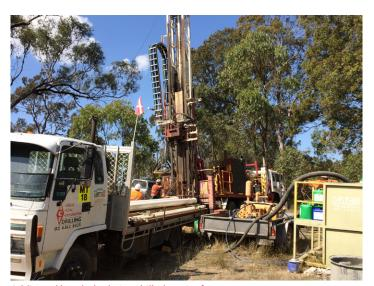
Additional boreholes being drilled on site for groundwater sampling and monitoring.
