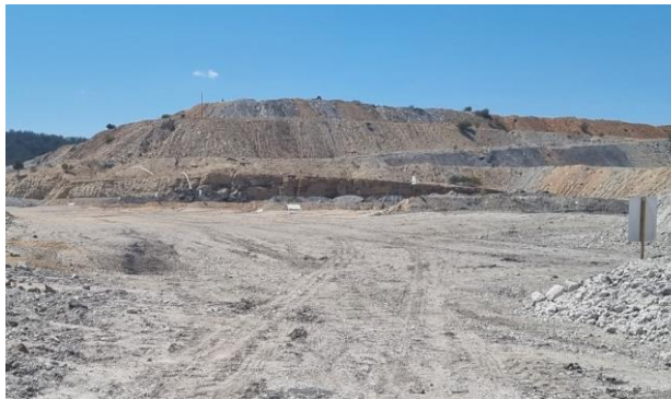
Photograph 10: Contaminated land remediation
