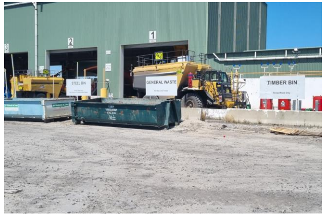
Photograph 5: Segregated waste storage
