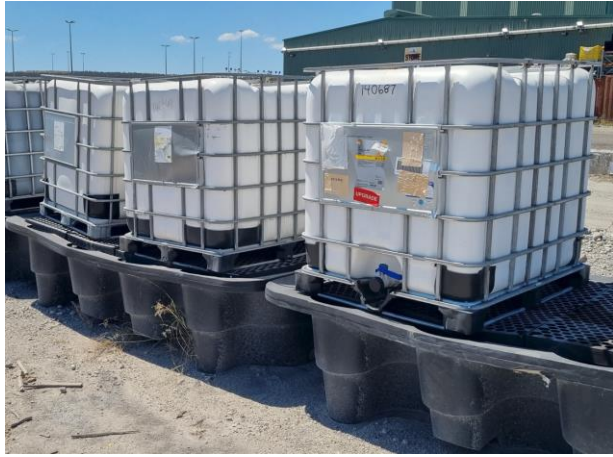
Photograph 6: Liquid storage on bunds
