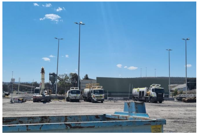
Photograph 15: Lighting directed below the horizontal
