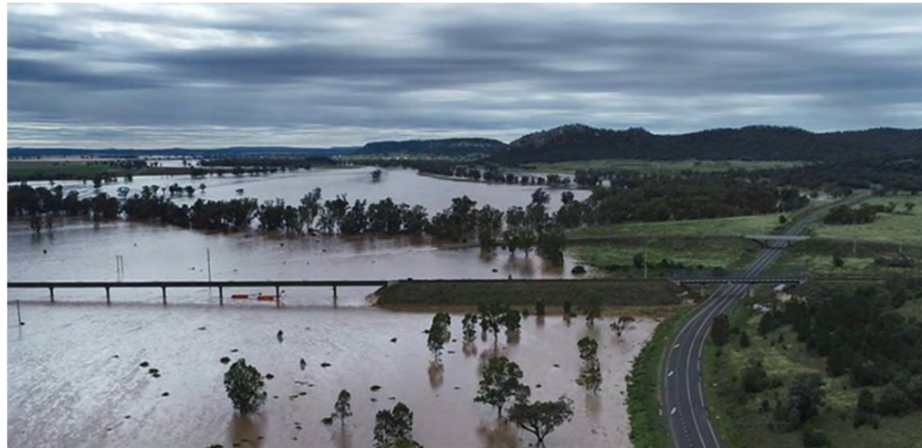
Namoi River – Kamilaroi Highway looking South
