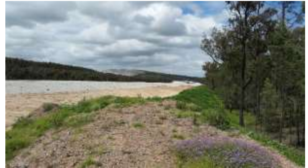
Photo 2 An example of the haul road, looking south
