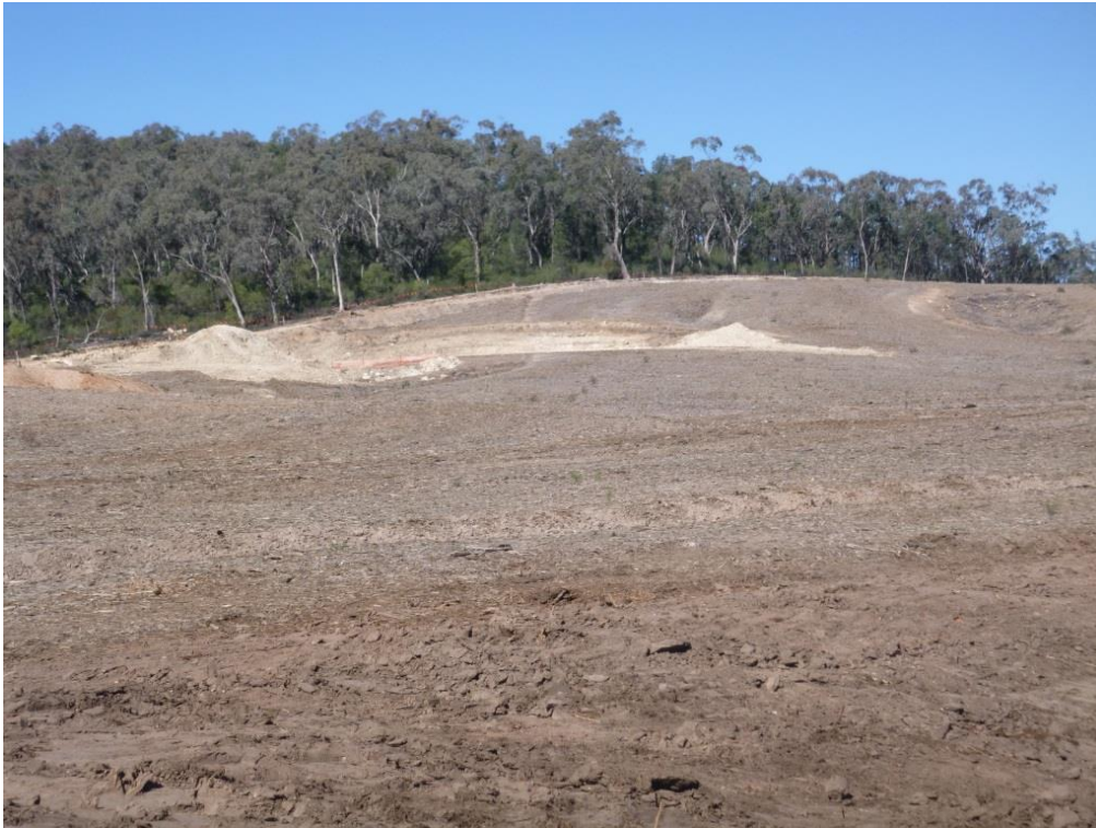
Photo 3 – Cleared area for rehabilitation
