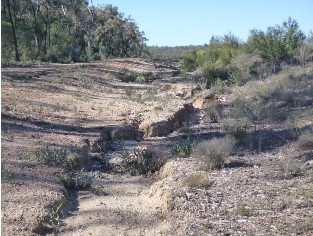
Photo 7 – Eroded section of a clean water drain
