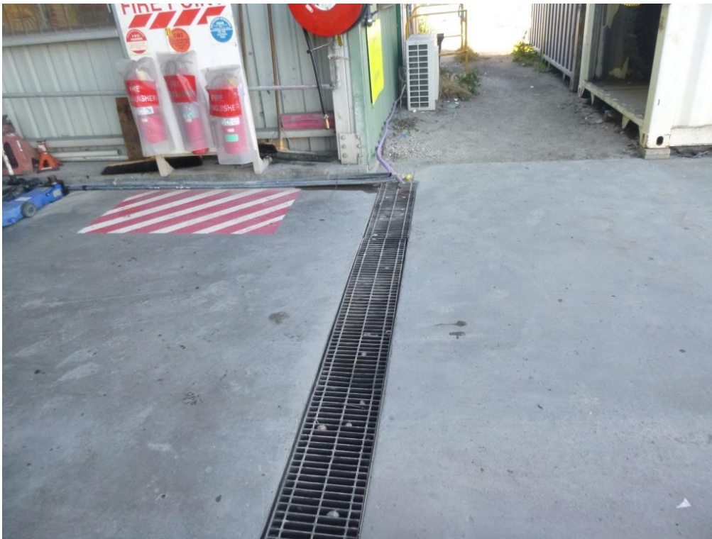
Photo 12 – Drain collects potential runoff from workshop area
