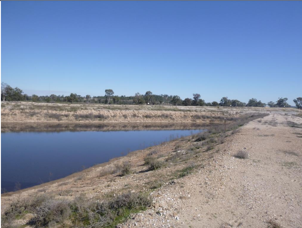
Photo 17 – Dam at TLO Area with large rilling
