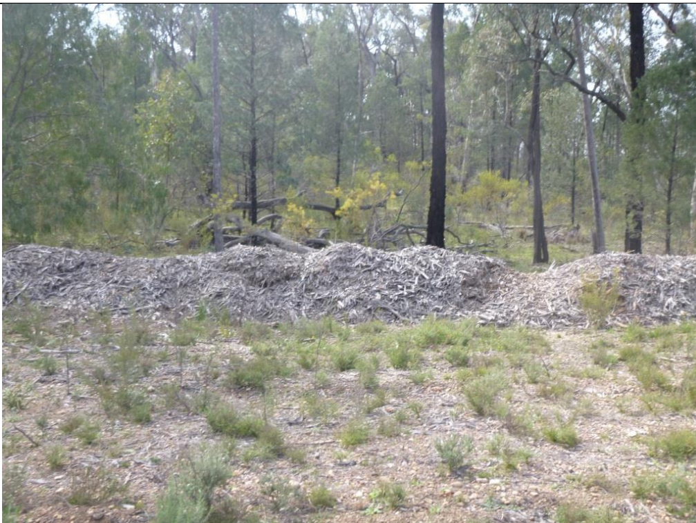
Photo 22 – Mulch has been used as an erosion and sediment control
