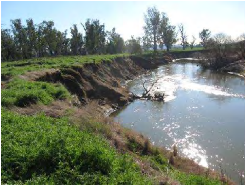
Photo E-19 Erosion along the banks of Namoi River
