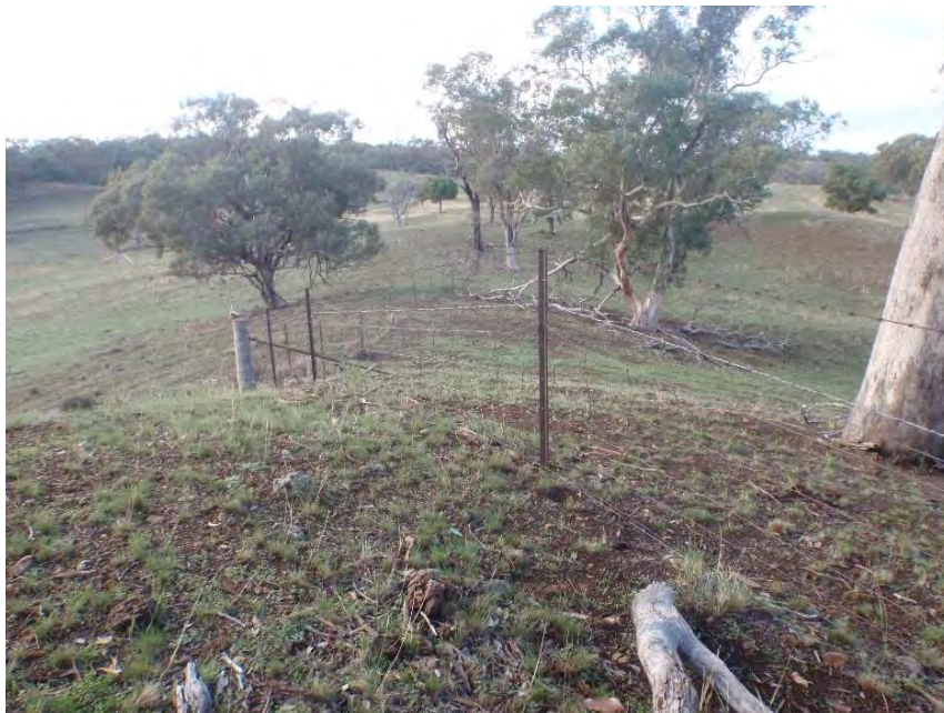
Photo E-3 Existing fencing which requires upgrades at Braefield
