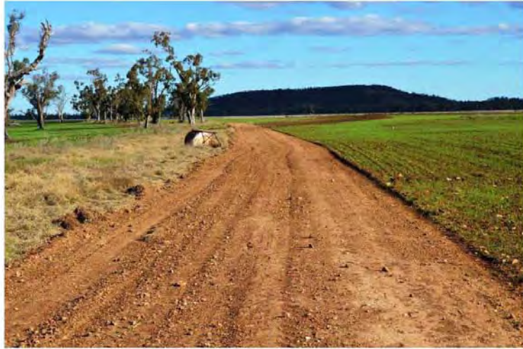
Plate 7 Roma Bore Hole and Pipeline facing South showing Warner's Road
