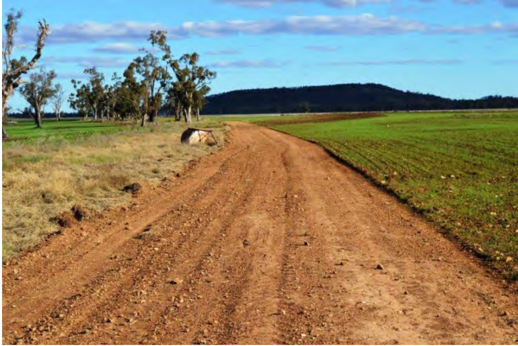
Plate 5 Roma Bore Hole and Pipeline Inspection Area Facing South
