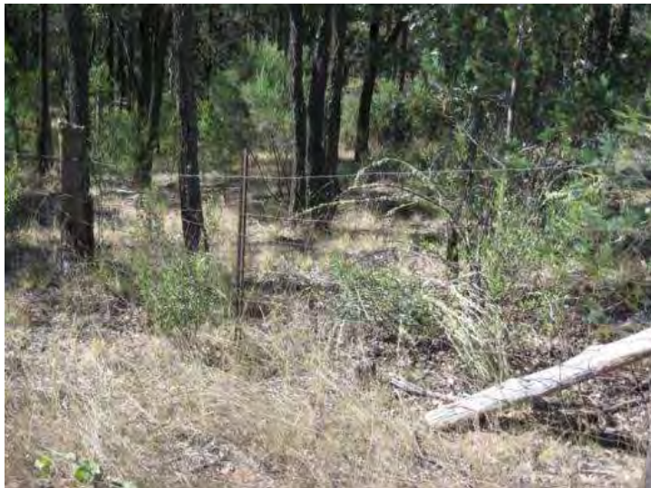
Photo 6.15 An example of existing fencing to be upgraded
