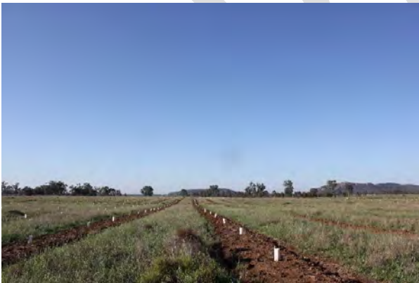
Photo 5.3 An example of 2018 restoration works completed in the Namoi BOA
