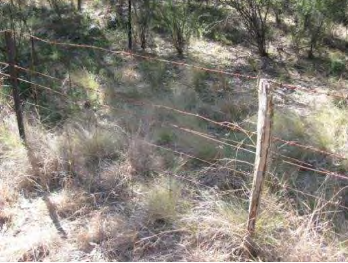
Photo 6.12 An example of existing fencing to be upgraded
