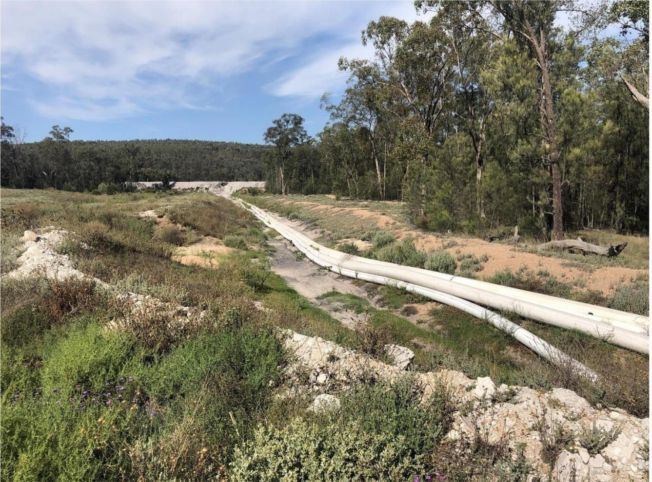
**Photo 18** Water pipelines noted to be contained within drainlines.
