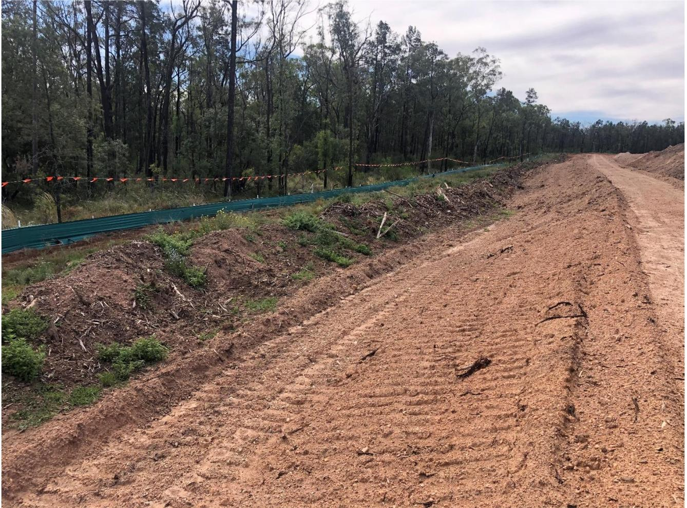
**Photo 21** Erosion and sediment controls at disturbance limits.
