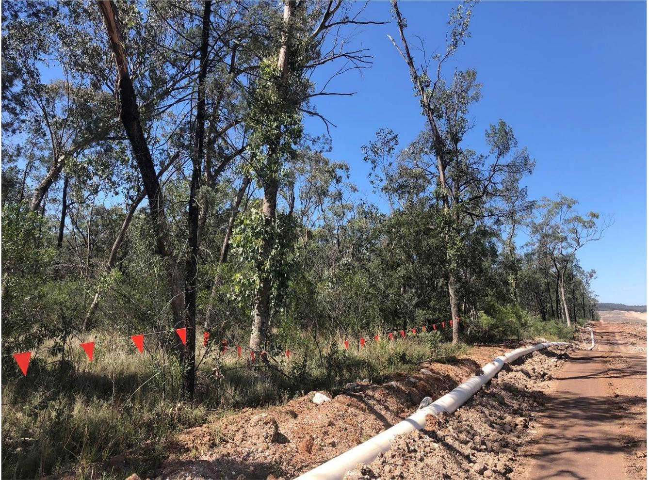
**Photo 24** Clear demarcation of disturbance limits. Pipelines contained within the site by bund.
