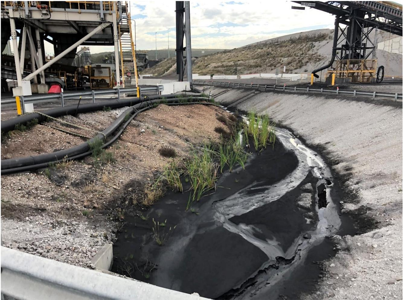
**Photo 7** Dirty water management system including pipelines in drains
