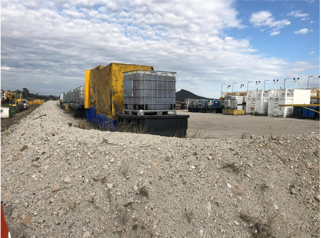
**Photo 15** Liquids storage in bunded containers and bunded laydown area
