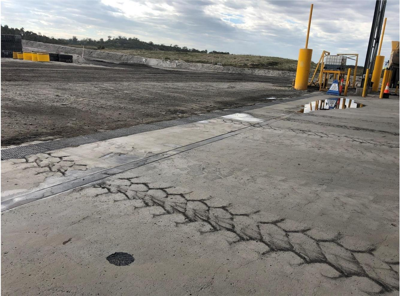
**Photo 10** Catch drain around boundary of workshop
