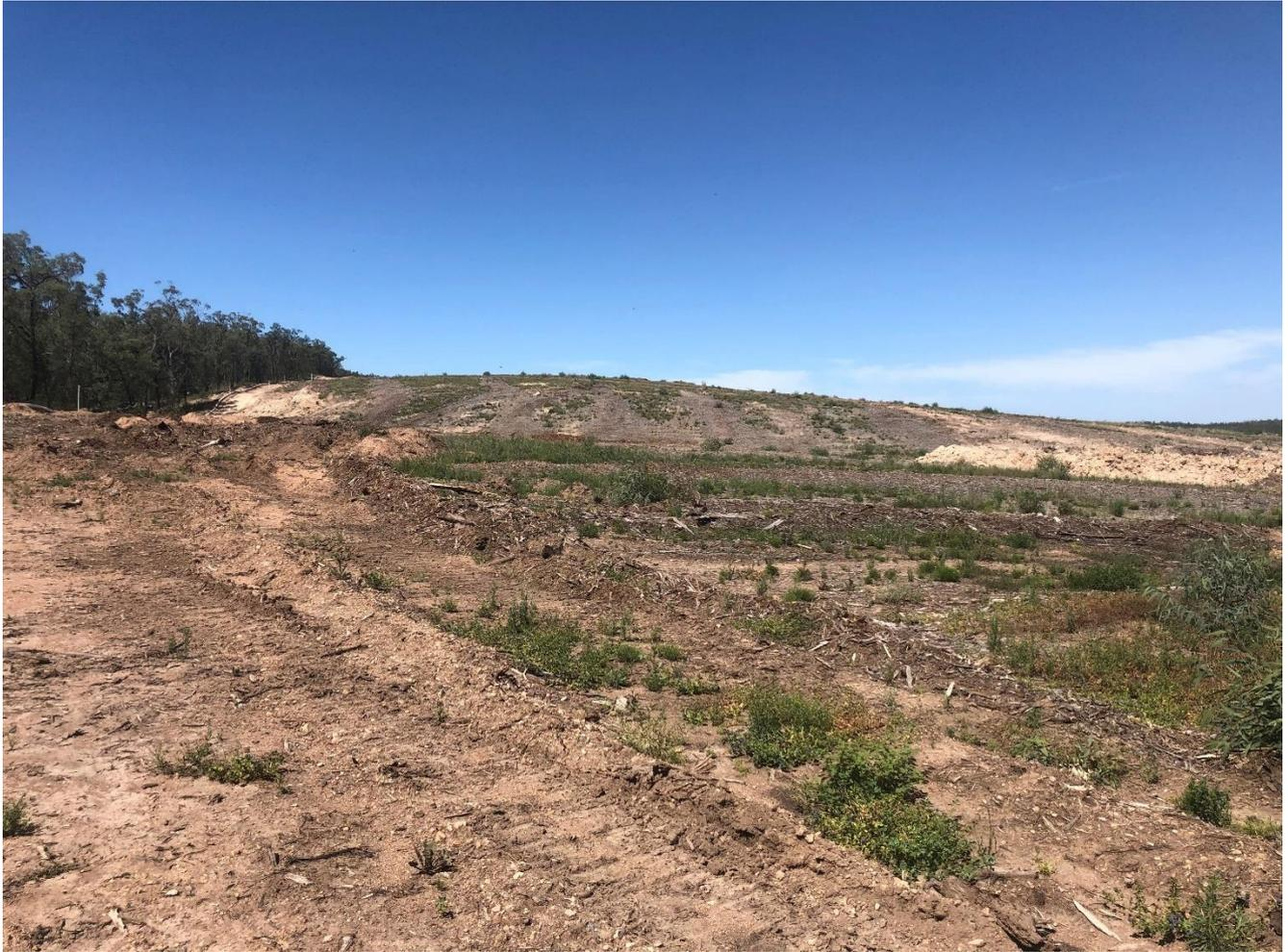
**Photo 23** Cleared and grubbed area ahead of mining
