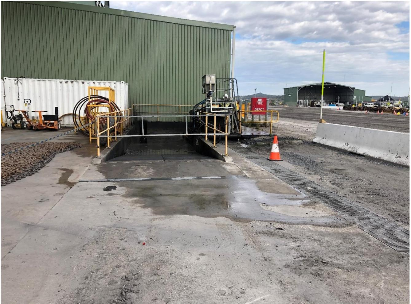
Photo 9 Catch drains in place reporting to sumps
