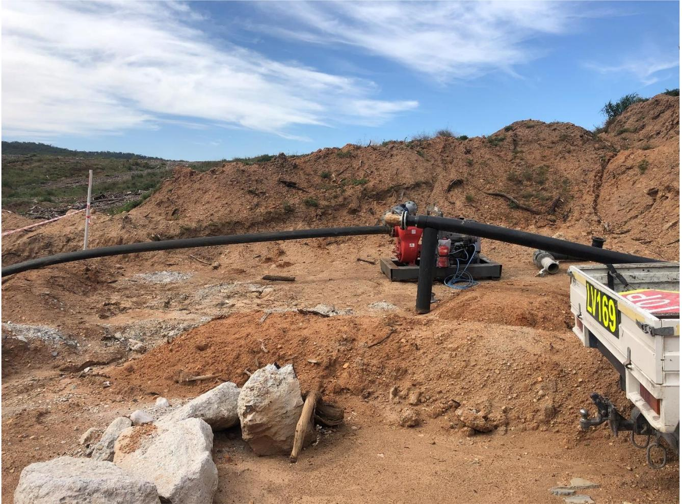
**Photo 20** Temporary bunding in place at remote pump
