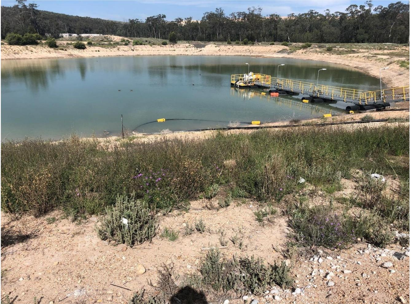
**Photo 19 Sediment dam. Note some weeds evident in batters.**
