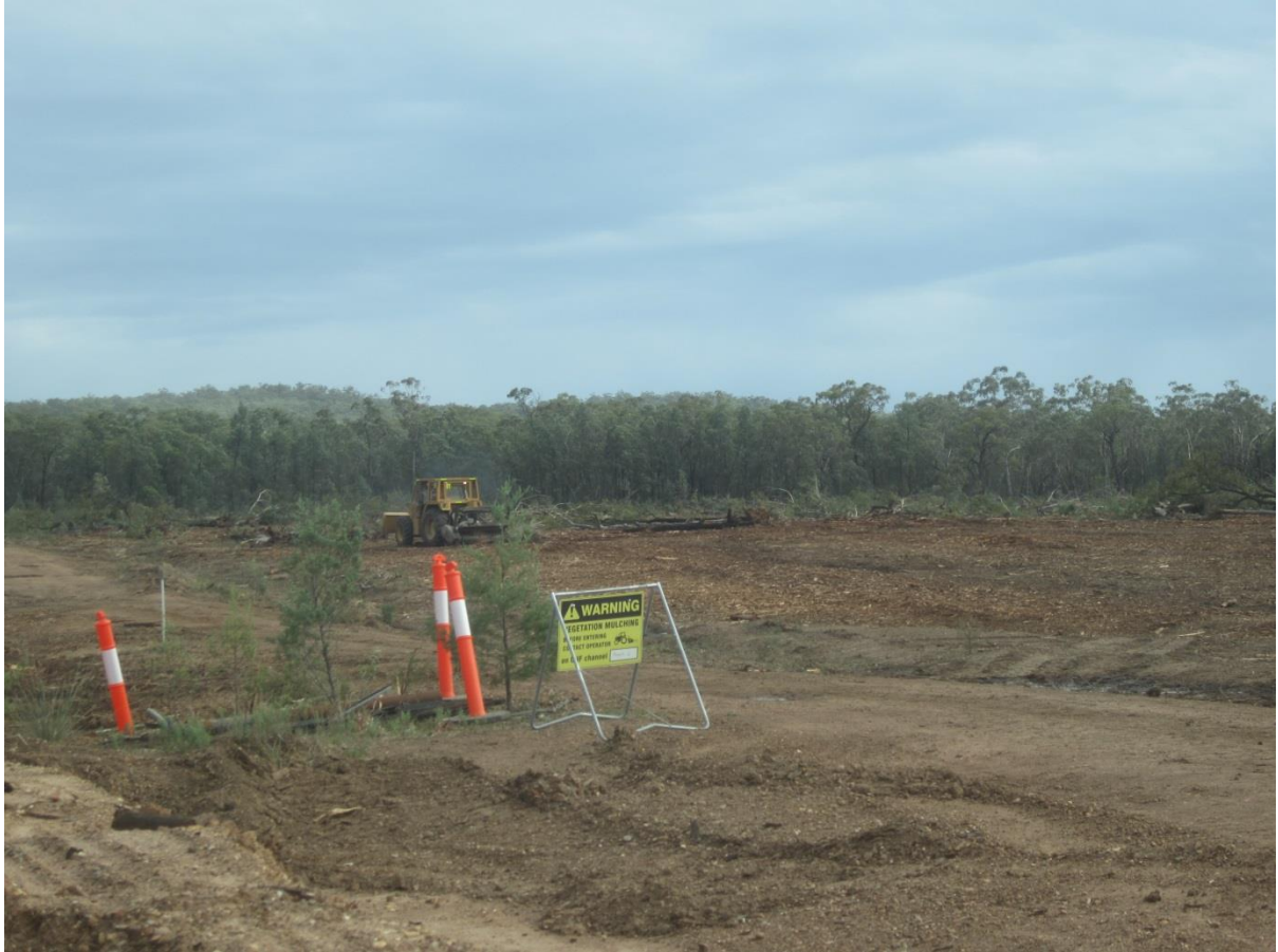
Photo 2 – Vegetation clearing – Stage 1 underscrubbing and grubbing showing signage
