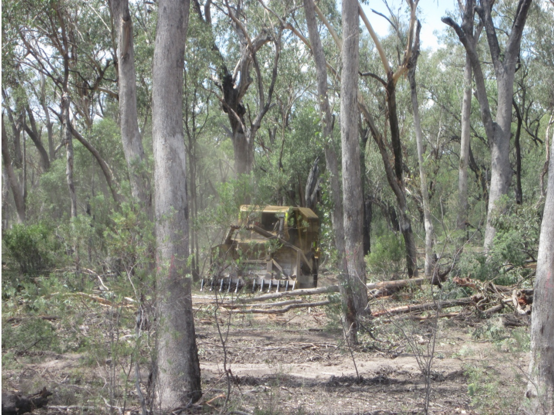
Photo 3 – Vegetation clearing – Stage 1 underscrubbing and grubbing showing marked habitat trees
