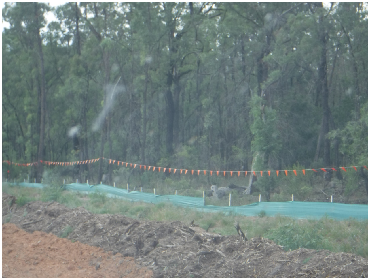
Plate 4 Example of delineation of clearing extent and fencing along biodiversity corridor and sedimentation capture fencing
