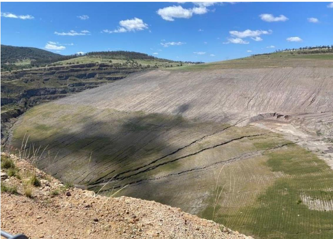
**Photo 6 – Extensive rilling and scouring in areas of completed rehabilitation in Open Cut 2**
