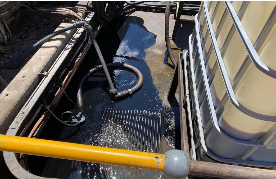
**Photo 10 – Drain blockage located in the fuel farm bunded area filling with hydrocarbon contaminated water**
