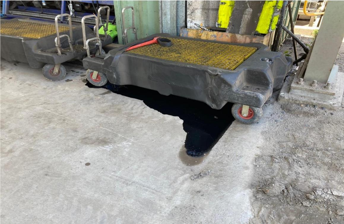
**Photo 9 – Unattended hydrocarbon spill located in refuelling area**
