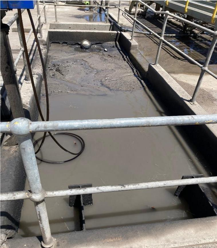
**Photo 11 – Oily water separator located near the wheel washing station appeared to be approaching capacity**
