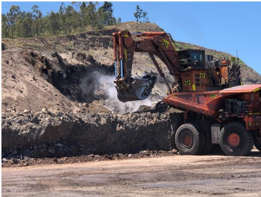
Figure 33: Photo of Spontaneous Combustion in previously dumped overburden
