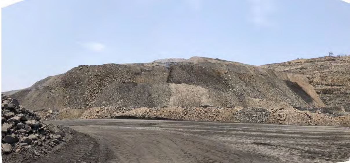
Figure 33: Photo of Spontaneous Combustion Management on Western Side of OC1 dumps
