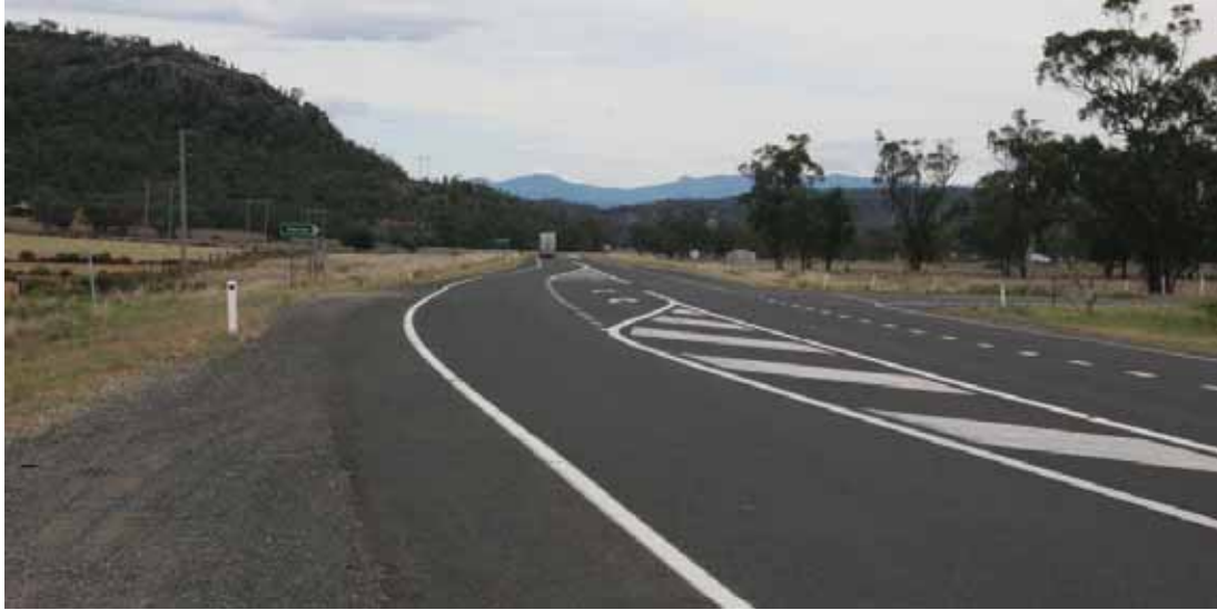
Photo 2-1 Kamilaroi Highway, looking northbound in the vicinity of the intersection with Manila Road to the right
