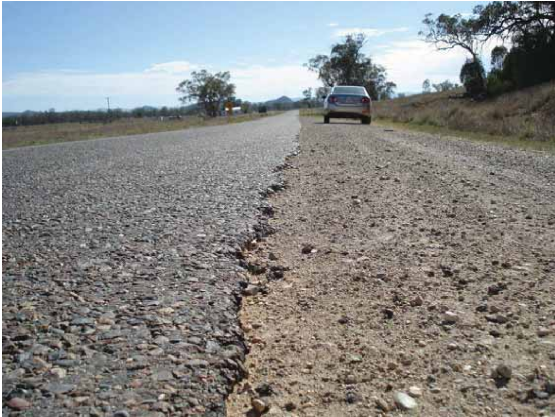
Photo 5 The edge drop-off, southern side of Manilla Road on the approach to the Kamilaroi Highway
