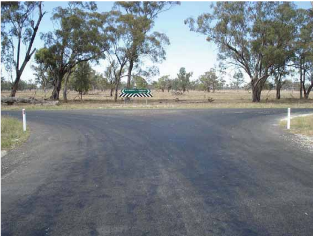
Photo 12 Faded centreline marking at the Manilla Road/Leard Forest Road intersection
