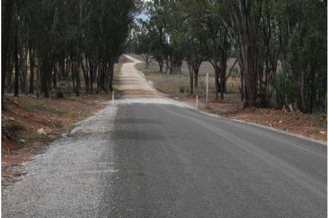
Photo 2-6 Goonbri Road, looking eastbound, approximately 200 m east of its intersection with Leard Forest Road
