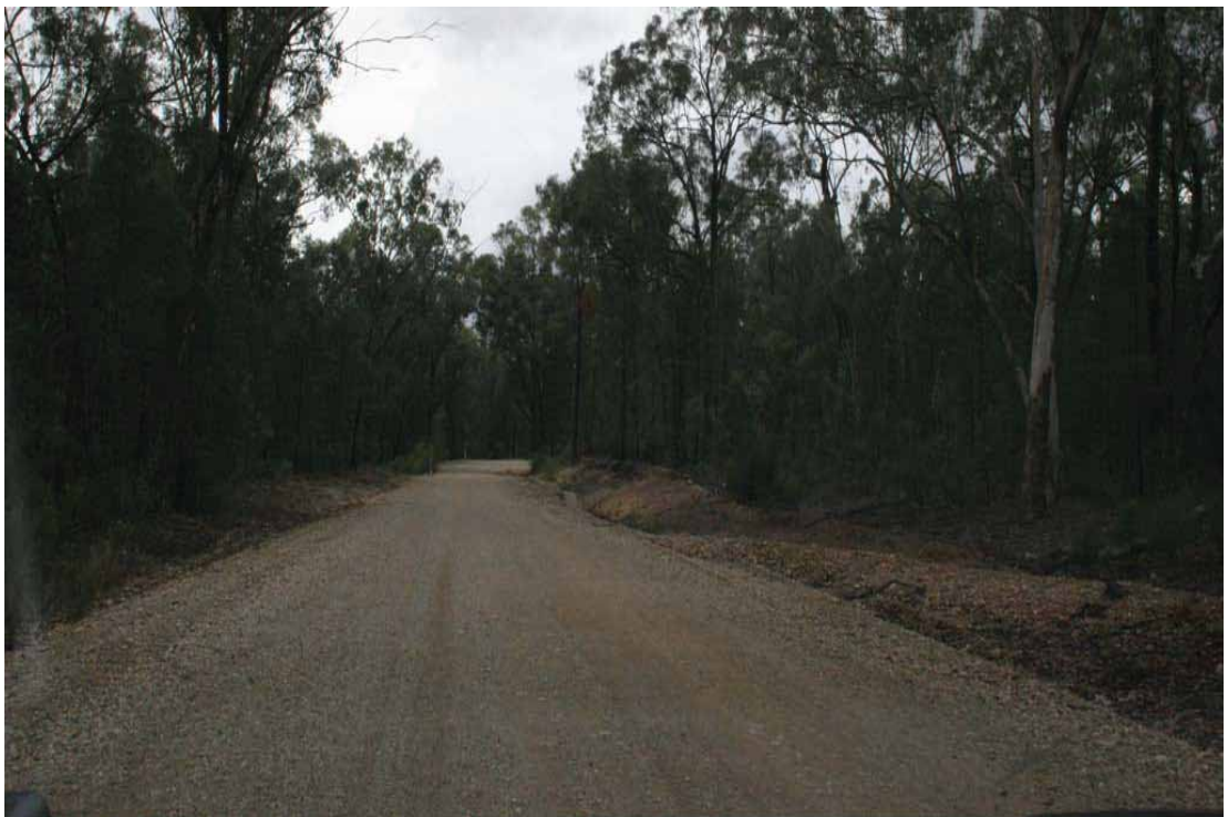
Photo 2-5 Unsealed rural road section of Leard Forest Road looking northbound
