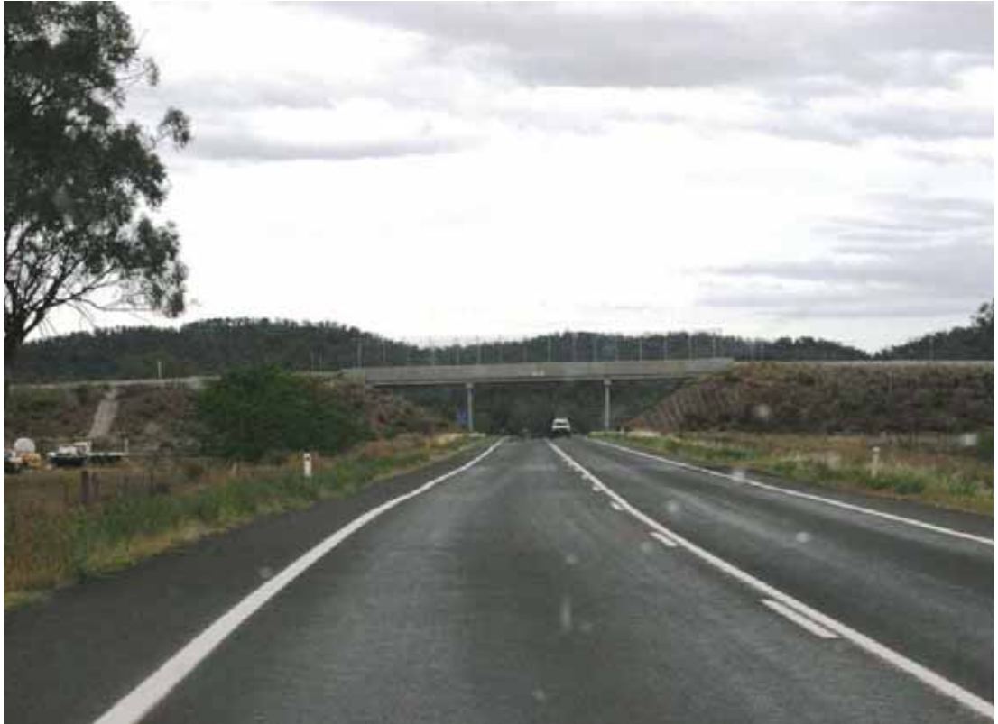
Photo 2-14 Boggabri Coal's private haul road crossing over the Kamilaroi Highway
