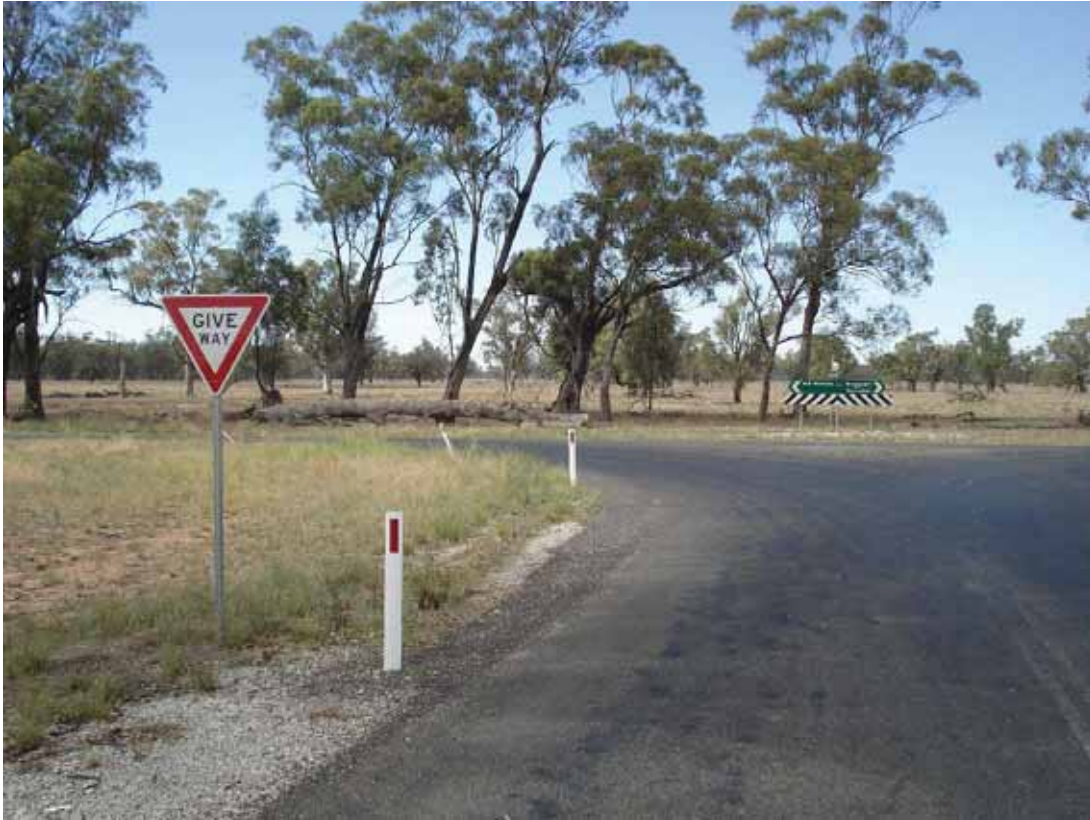
Photo 13 No give way line on Leard Forest Road
