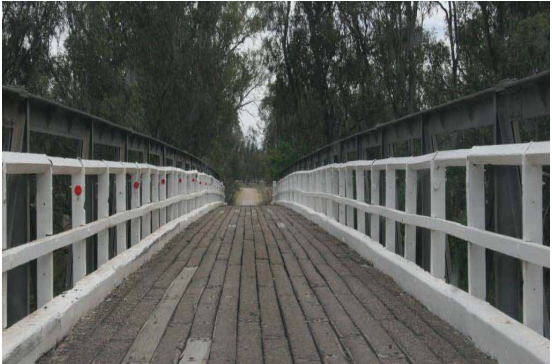
Photo 2-9 One-lane bridge on Harparary Road across Namoi River, looking westbound
