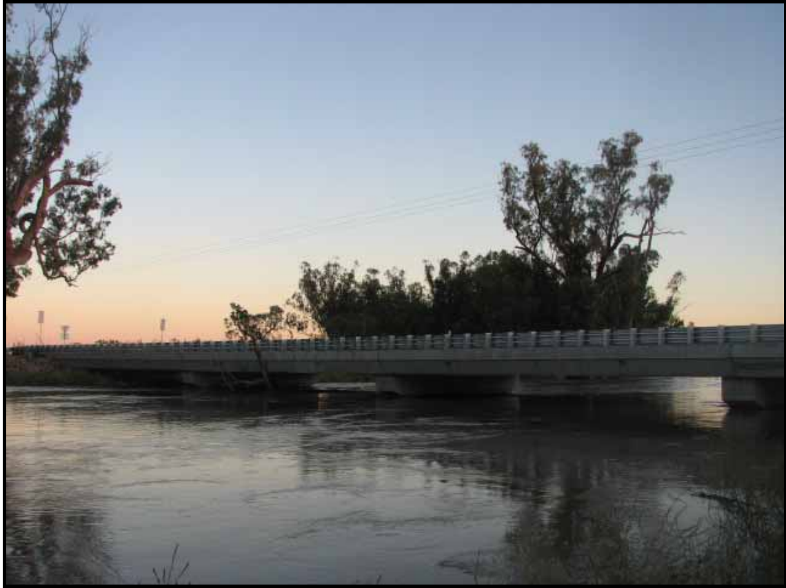
Figure 2.2 Boggabri Coal Haul Road Bridge during the Namoi River December 2008 Flood
