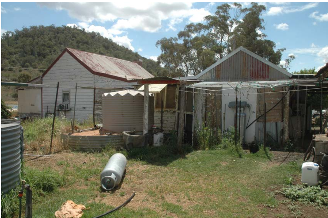
Figure 29 - Heathcliffe. View from south. Main residence to left, kitchen to right.
