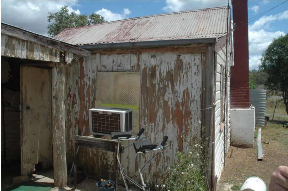
Figure 30 – Heathcliffe. Exterior of main residence. Note original slabs.
