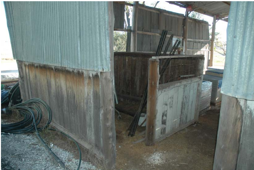
Figure 8 – Nagero 2. Southern wall showing timber cladding.
