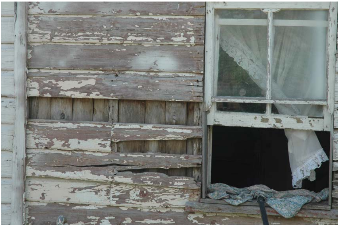
Figure 31 – Heathcliffe. Detail of exterior showing original slabs beneath weatherboards.
