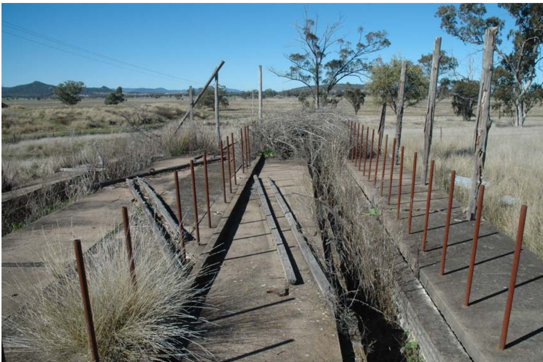
Figure 25 – Daisymede 3. View to east across farrowing shed floor.
