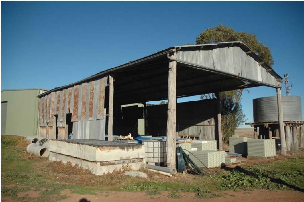
Figure 7 – Nagero 2. View from north-west. Note new shed to rear.
