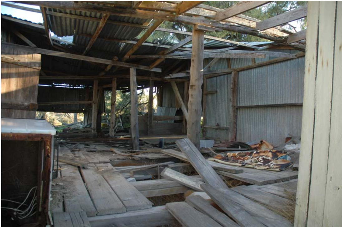
Figure 12 – Nagero 3 - Interior View
