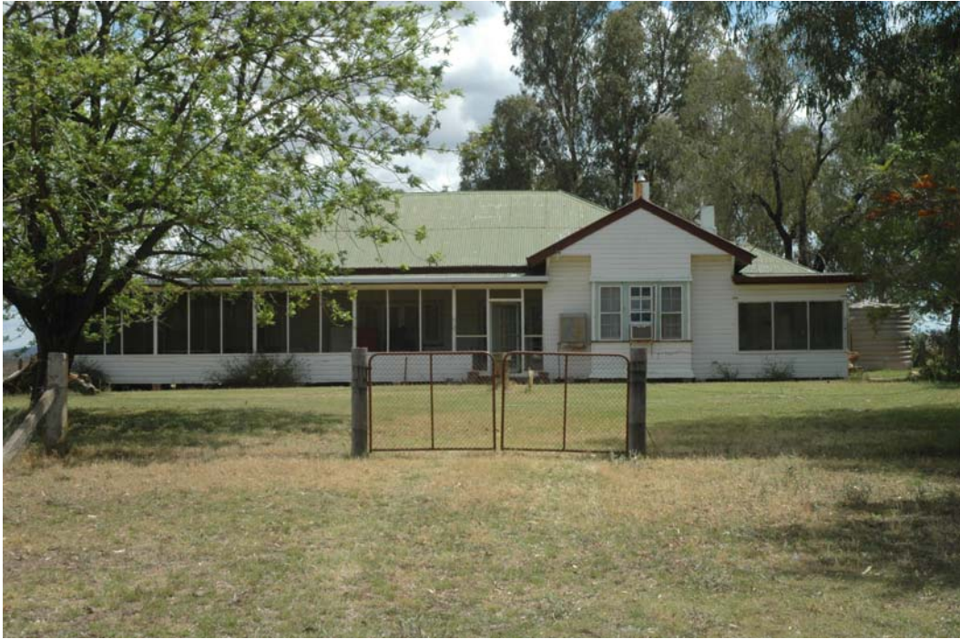
Figure 15 – Merriown. View to front of main house.
