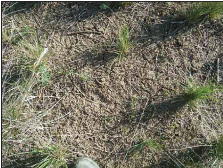
Plate 6 The high shrink-swell clays of the Namoi River floodplain – note the cracking of the surface soil.
