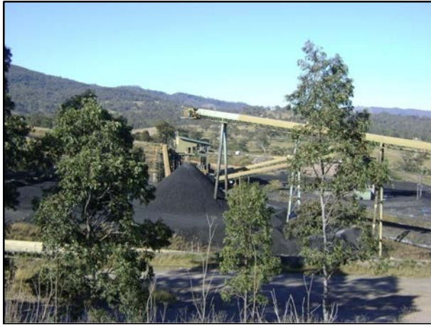
Figure 5 - COAL PREPARATION PLANT - crushed coal is reclaimed and processed in the CPP
