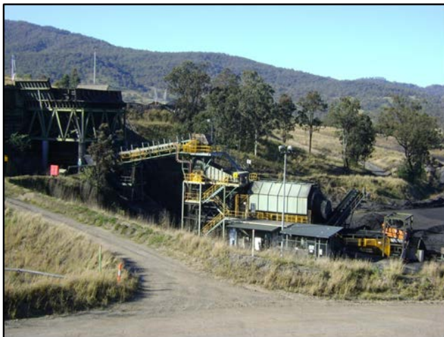
Figure 4 - COAL CRUSHING PLANT - coal is placed into a receival bin then fed into a rotary breaker
