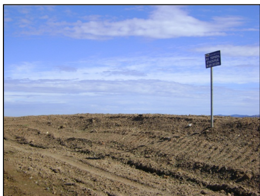
Figure 1 – SIGNPOSTED TOPSOIL STOCKPILE
